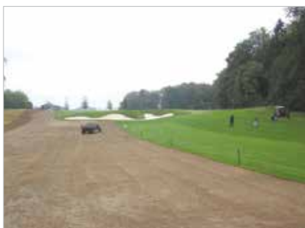
3rd Fairway renovation (October 2013)
